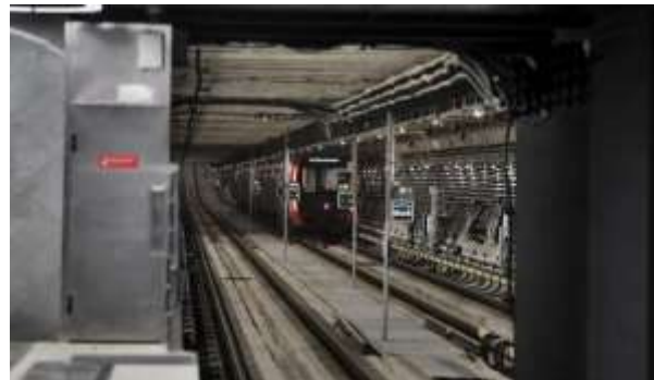
Fig. 2. Double track tunnel
